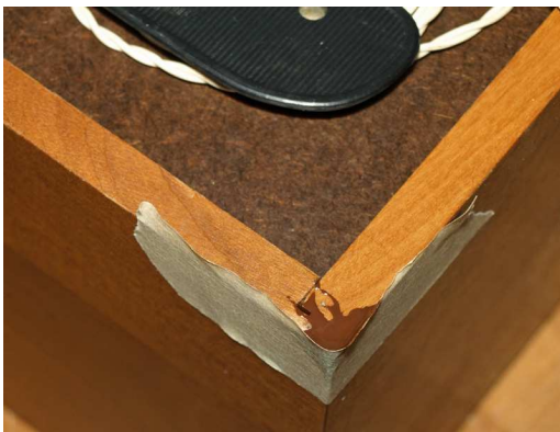
fig 11—corner bash, tape dam and epoxy filler
