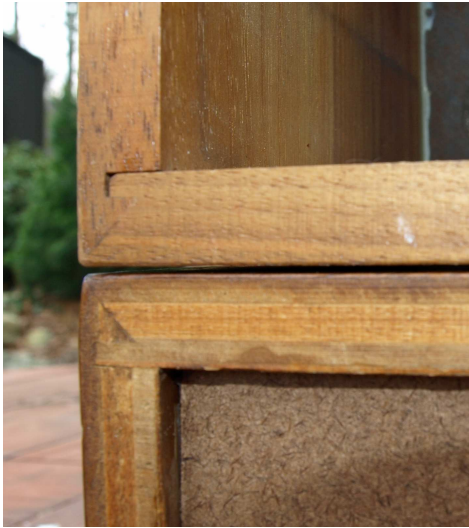
fig 5 --Veneer (bottom) and solid (top) cabinets
